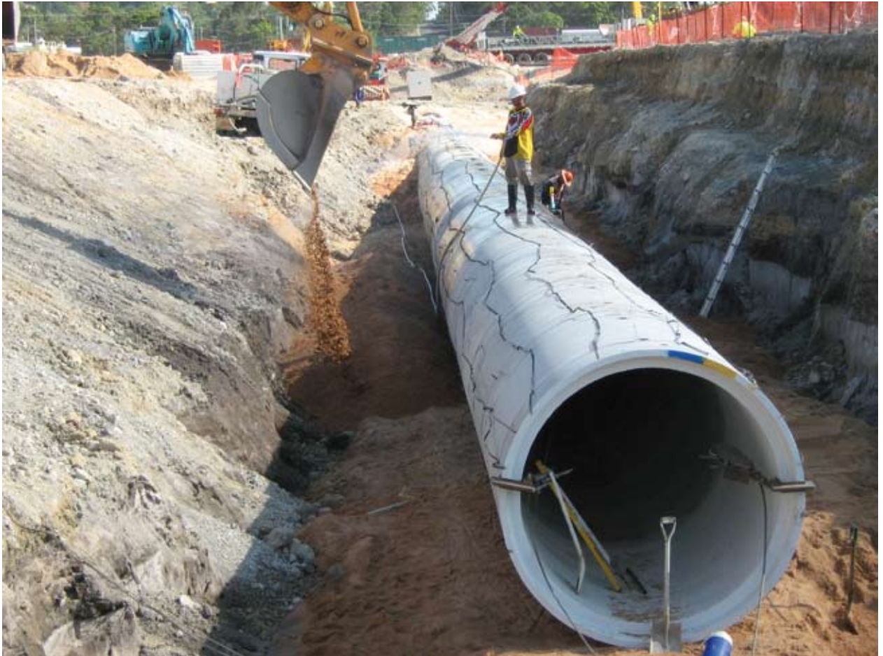
Tugun desalination project construction
